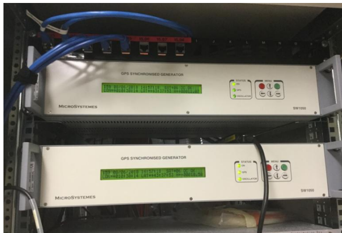
GPS synchronized 10 MHz timing generator
