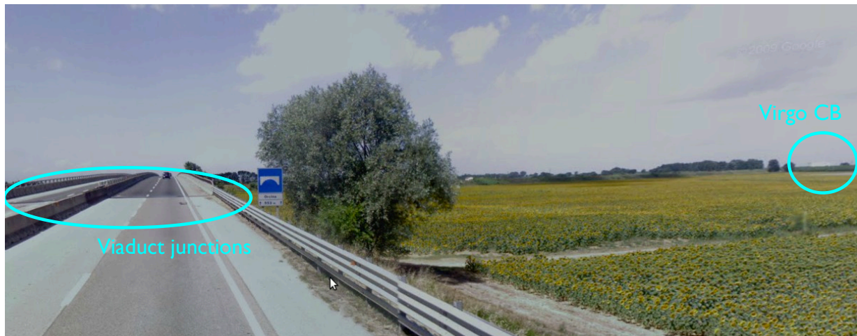
Figure 14: Snapshot of one of many viaduct junctions hit at the passage of trucks. The junctions are the most likely origins of the antropoc seismic waves reaching the Virgo site from the southern direction (in the picture at the extreme right).
