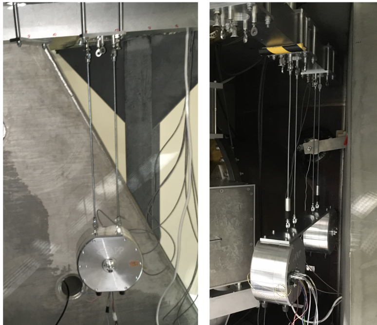
Figure 1: The left picture shows one NCal-200 suspended on the north side of the north end tower. The right picture shows two NCal-200 suspended from the same support plate on the south side of the north end tower
