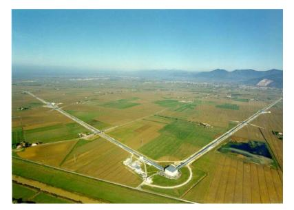
Aerial view of the Advanced Virgo site in the vicinity of Cascina, near Pisa, in Italy. The upgraded interferometer will use the same Virgo infrastructure, at EGO (European Gravitational Observatory), consisting of two 3 km long arms and several buildings in the central area and at both arm ends.
